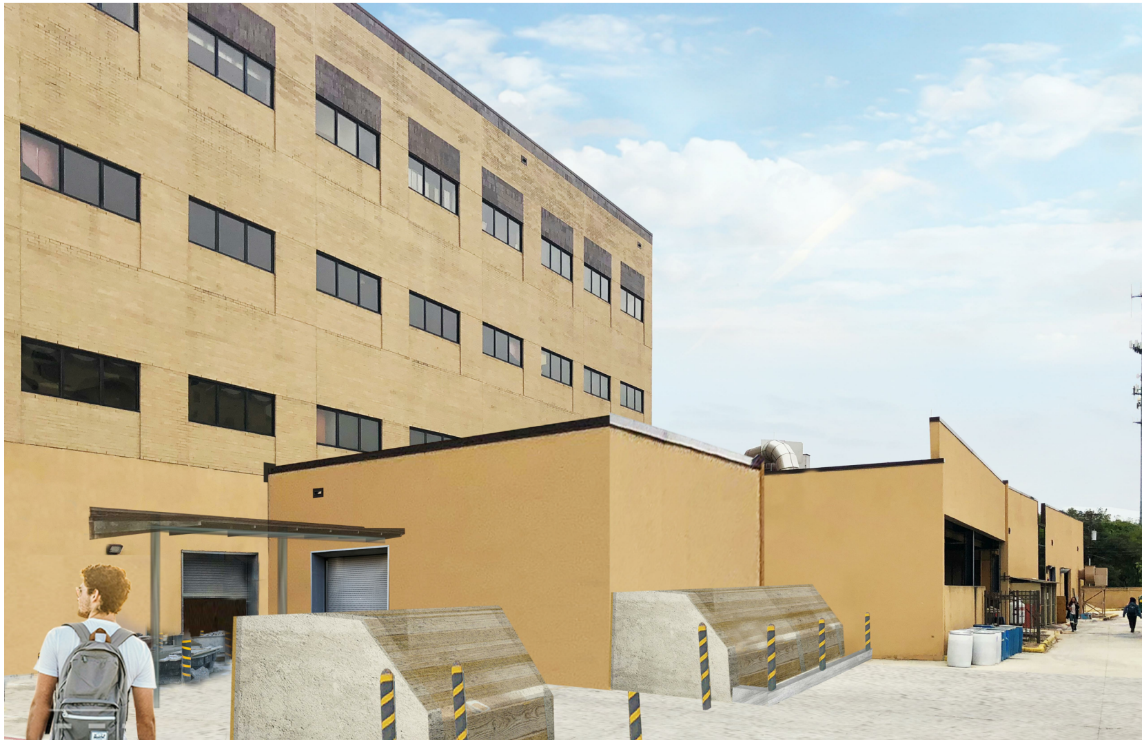
PERSPECTIVE - VIEW OF SOUTH AND EAST FACADES TEXAS STATE UNIVERSITY | R.F. MITTE ENGINEERING BUILDING SPACE RECONFIGURATIONS
